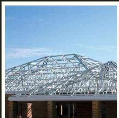
SCG Roof TRUSS
